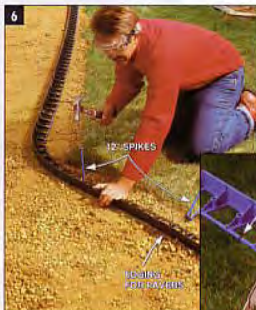
6 12" SPIKES 10" WEBBING FOR PAVING CUT INSTALL THE EDGING on the tamped subbase using 8" - 10" spikes. Cut the webbing on the edging's back side to make it flex for curves.
