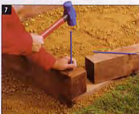
6 12" SPIKES 10" WEBBING FOR PAVING CUT INSTALL THE EDGING on the tamped subbase using 8" - 10" spikes. Cut the webbing on the edging's back side to make it flex for curves.
